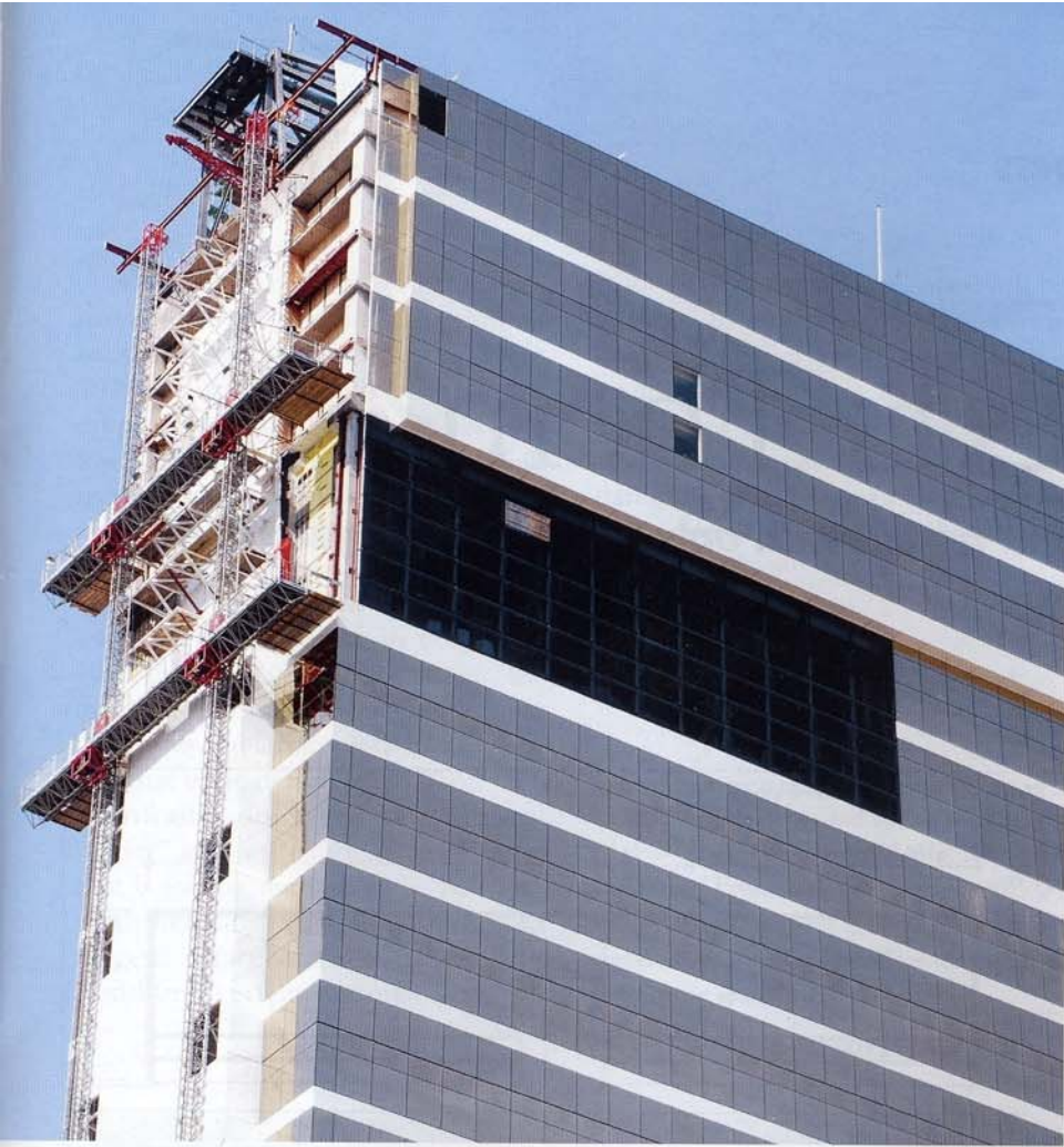
A dual twin, two units stacked on top of each other, sharing a common mast was used.
