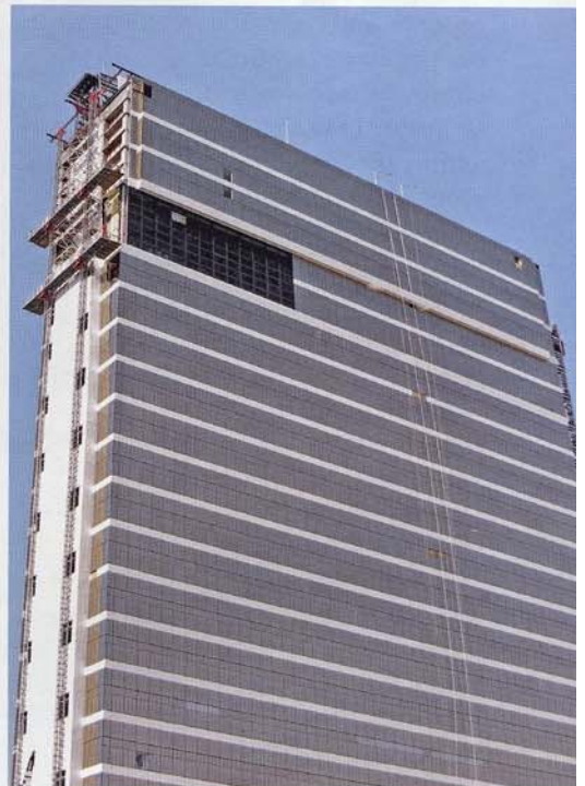
Strong wind conditions made the job a challenge.
