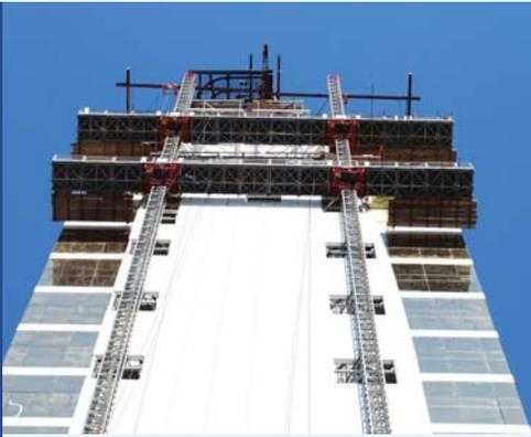
After a fire destroyed the south side of the **Borgata Hotel & Casino** (above), NEMC provided a solution of a dual twin on one set of mast to expedite the completion, allowing two contractors to work on demolition of the damaged panels/curtain wall at once.
