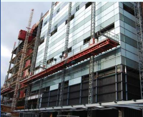
**The Wexford Science Center** (above) required the use of nine units to perform the installation of curtain wall systems. This is a typical project in size and scope for NEMC. Engineered drawings were required for each unit and a layout for where the units were to be positioned on the building.
