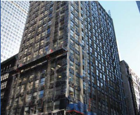
Equipment was used to install a curtain wall system to re clad the entire building of **1140 Avenue of the America's** (above). This project had multiple contractors working on the mast climbers. The location of this project, one block from Time Square, made it a challenge with the amount of pedestrians and vehicle traffic on the street.
